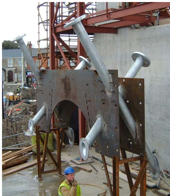
Figure 8 Pylon Head Steel Assembly
