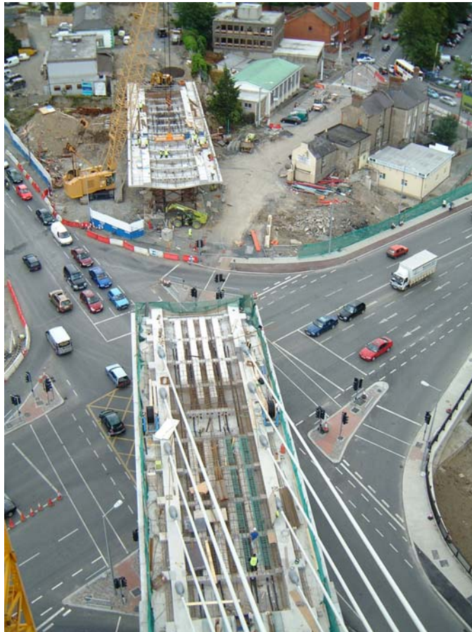
Figure 17 Bridge during Segment Erection
