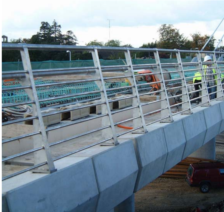
Figure 12 Stainless Steel Parapet
