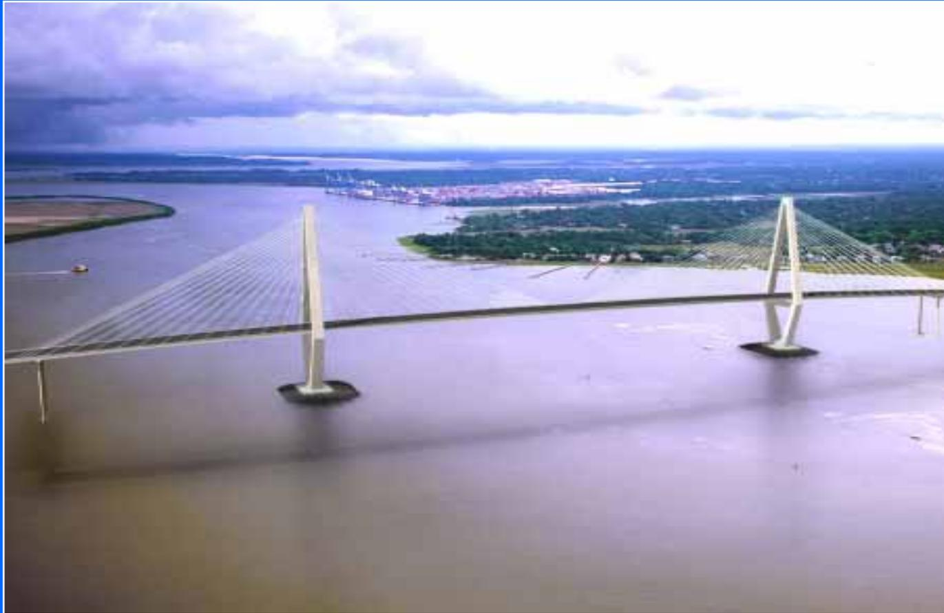
**The new bridge has steel edge girders and floor beams. The total bridge length is 13,200 feet (2.5 miles) end to end.**
